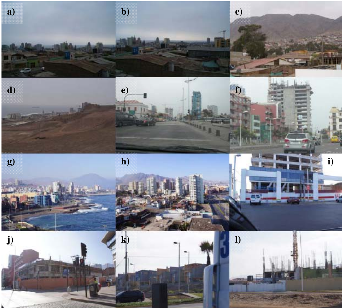
Figure 5. Pictures from site-visits in Antofagasta: a) south-west side, b) west side (coastal), c) east side, d) view of the shoreline from residential south side, e) typical shoreline, f) typical construction of residential high-rise reinforced concrete shear wall building, g) panoramic south view of the coast line, h) panoramic view of downtown, i) typical reinforced concrete frame systems, j) low-rise reinforced concrete building in downtown, k) new residential reinforced concrete buildings, l) typical construction of low-rise buildings in residential areas in the north side.
