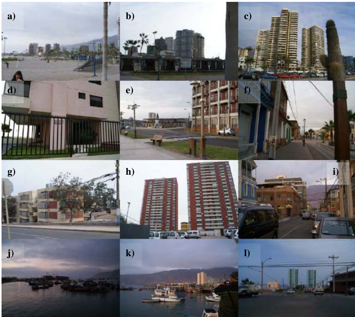
Figure 4. Pictures from site-visits in Iquique: a) North view of main beach (Cavancha) and buildings, b) south view of buildings in the shoreline, c) typical high-rise reinforced concrete shear wall buildings, d) first level of a 20-storey building next to main beach, e) main entrance from the coast to the historic downtown of Iquique, f) typical heritage wood buildings in downtown, g) south part of Iquique showing typical confined masonry shear wall residential buildings, h) mid and high-rise buildings in the south-west side, i) historical buildings near the ports, j) view of fishing boats and main port of Iquique, k) west north side with a view of the coast and nearby buildings, and l) view from a safe zone in the south side.
